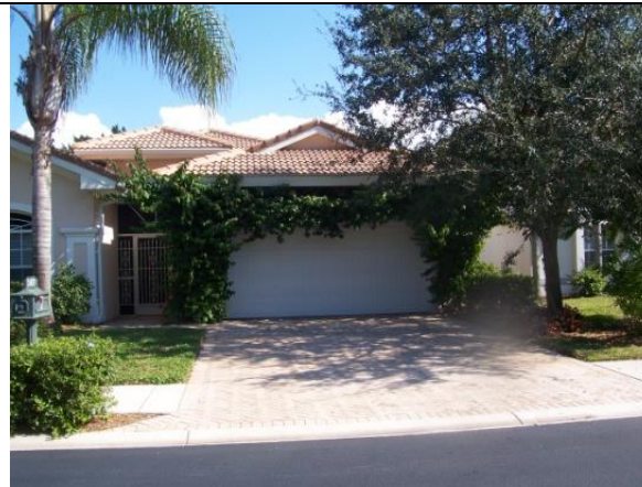
Bougainvillea over garage door needs pruning
